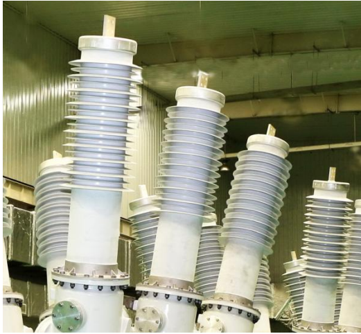
Compound insulating bushing
